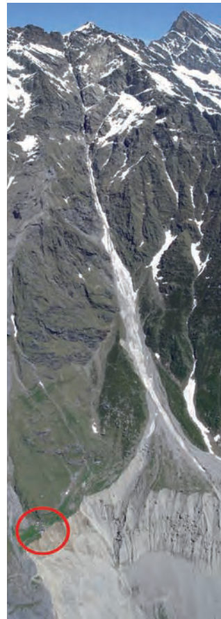
Figure 5 (left): Slope at Mettenberg near Grindelwald after a landslide. The hut (red circle) was also destroyed by the slide.
