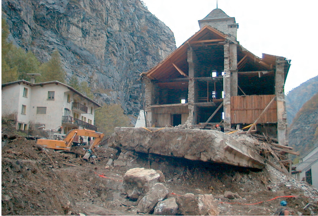
Figure 2: Mudslide in autumn 2000 in Gondo, Valais, after heavy precipitation. (Source: Union of cantonal fire insurances, Commission for natural hazard damage prevention. VKF, Bern)
