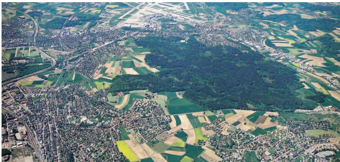
Figure 2: Large-scale photograph with Kloten, Wallisellen, Opfikon, Hard (2004): The web-like structure between the municipalities is clearly visible (Source: Swiss Air Force).
